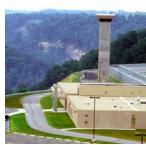
Correctional Facilities Big Sandy United States Penitentiary and Prison Camp, Inez, KY
