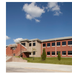
Barracks and Housing Starship Barracks Renovation and Dining Facilities, Ft. Jackson, SC
